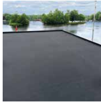
40.9991 EPDM roof covering 1.14mm thick, to specification per m 2
